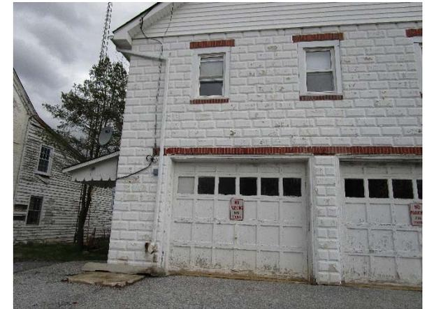
Downspouts along the building can lead to cisterns. Collected stormwater from the cisterns can be used to wash emergency vehicles or for other non-potable purposes. A preliminary soil assessment suggests that the soils have suitable drainage characteristics for green infrastructure.
